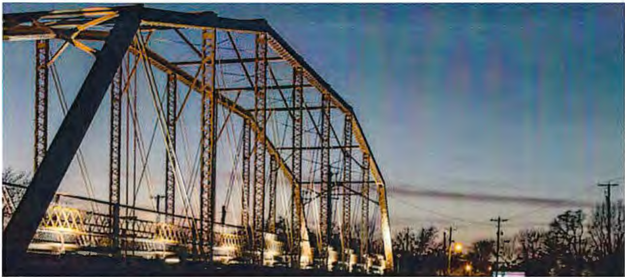
Figure 30: Photograph of the Kitzelman Bridge 55
