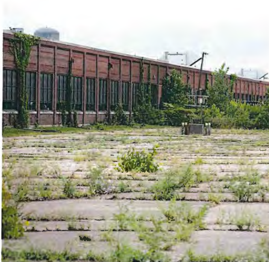
Figure 5: Former Borg Warner Site 13
