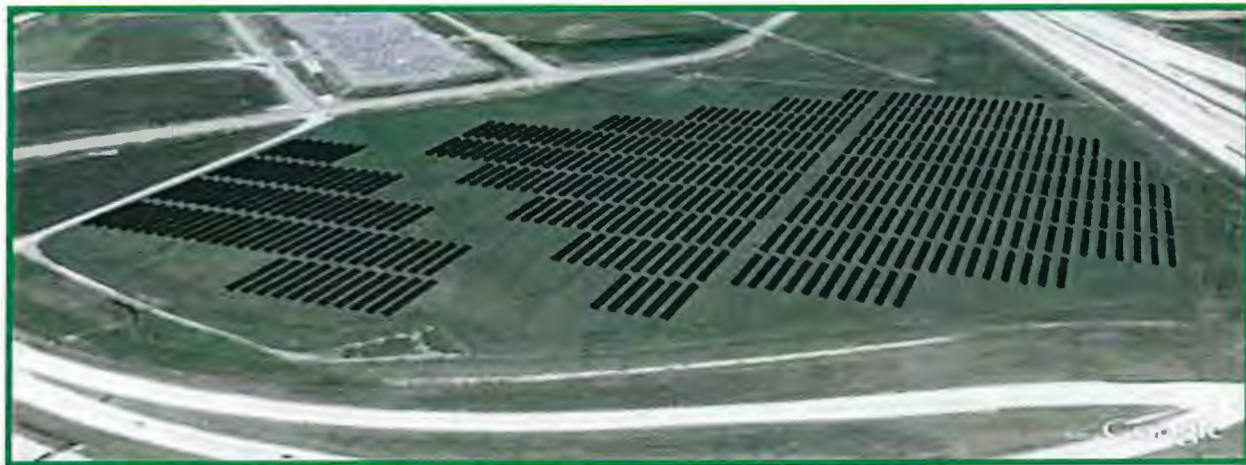
Figure 18: Indianapolis Airport solar farm 37
