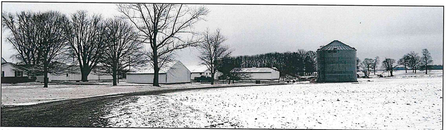
View of the site from CR 850 W looking northeast. This view shows the part of the residential structure on the left-hand side and the agricultural structures on the site.
