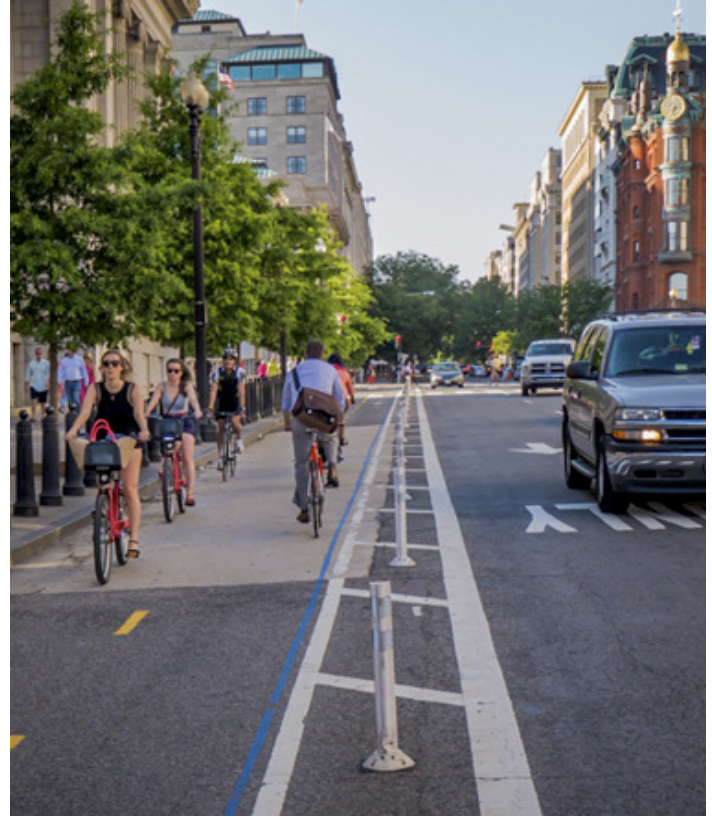
Two-way protected bike lane - How to Build A Great Menlo Park Bike Network, Oct. 2016
