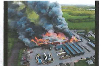
Major fire at solar-powered warehouse ... pv-magazine.com
