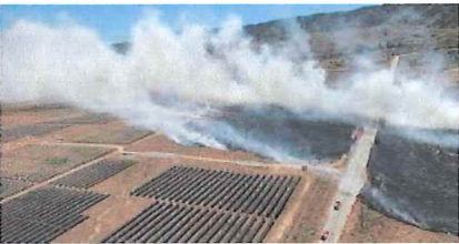
Brush fire at solar generating facility ... wildfiretoday.com
