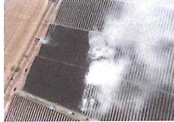
Finley solar farm fire ... sheppnews.com.au
